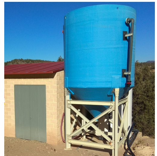
THE SMALL PLANT: View of the small plant with the sedimentation tank outside.
