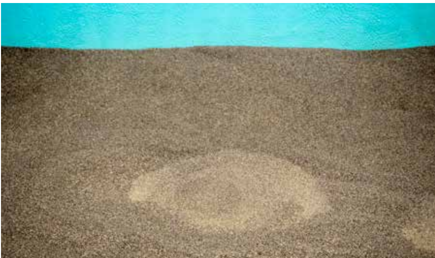
Nitrification and denitrification filters at VEAS use Filtralite products as media.
